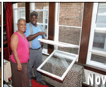
GADC partnered with GRANDFamilies: Generations Creating a Legacy, the City of Chicago Department of Aging, and Granville Love, proprietor of Team Construction, to install new windows, fascia and screens in Alma Donald's home—a senior and Englewood resident.
